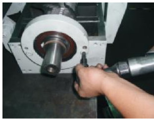
Picture 3-5: Installation of Bearing and Cutter Shaft 3
